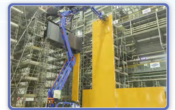
Workability verification and skill training related to Unit 2 R/B operating floor decontamination Training taking full advantage of the height of the Full-scale Mock-up Test Building and using water in an environment similar to the actual site
